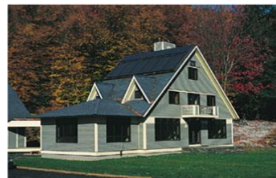
(b) Luxury home solar panel application
