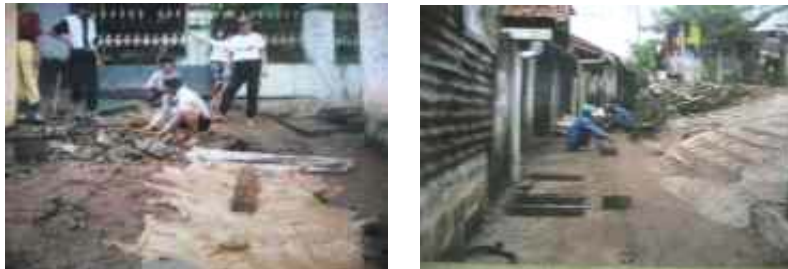
Figure 5. Construction of Local Street by the Community Source: Field Observation
