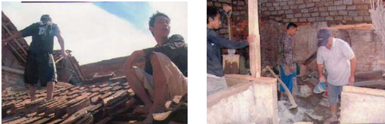
Figure 4. Renovation of a Poor-Condition House by the Community Source: Field Observation
