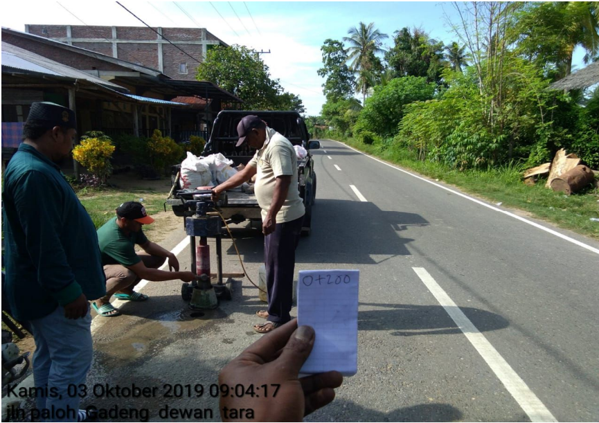
Gambar 4.20 Core Drill Sta 0+200
