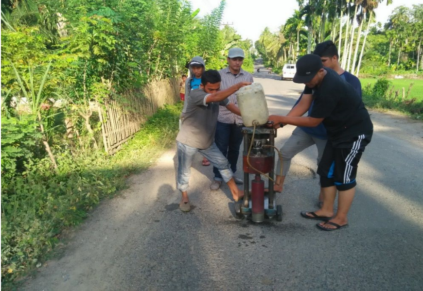
Gambar 4.12 Persiapan core drill benda uji
